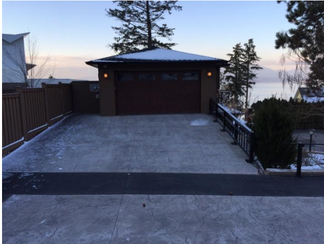
Subject Property Photos: 4962 Lakeshore Road East Elevation (facing Lakeshore Rd)
